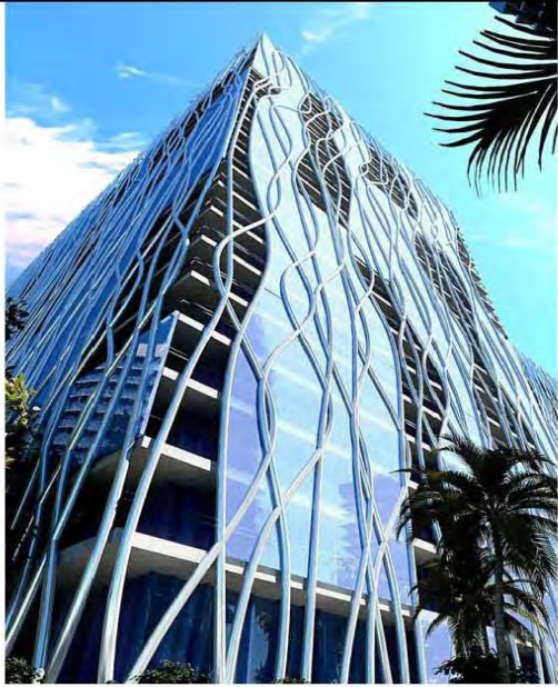
Latrinza Towers in Abu Dhabi, United Arab Emirates is a rectangular building decorated with pipes made of curved steel and use glass reflectors that provide a wonderful sight when they reflect sunlight. The towers consist of a set of four towers adjacent to each other.
