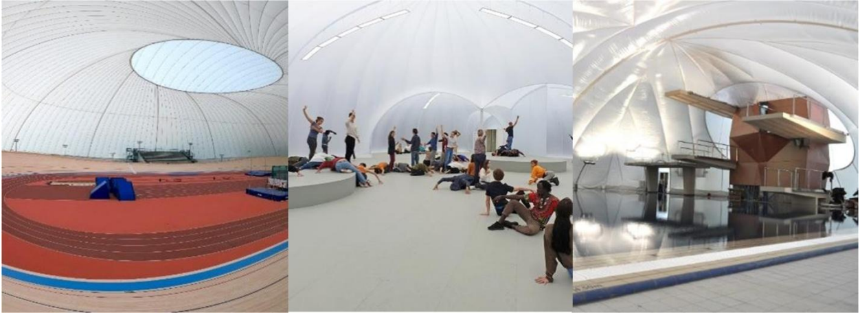
Figure 5: Air supported fabric based structures (Source: DUOL)
