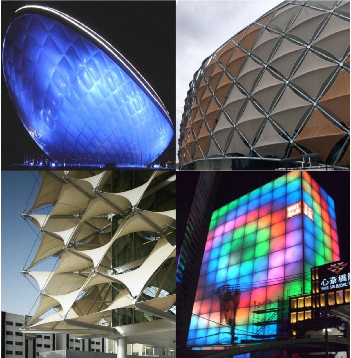
Figure 2: Advanced high performing fabric façade (Source: Taiyo Europe)
